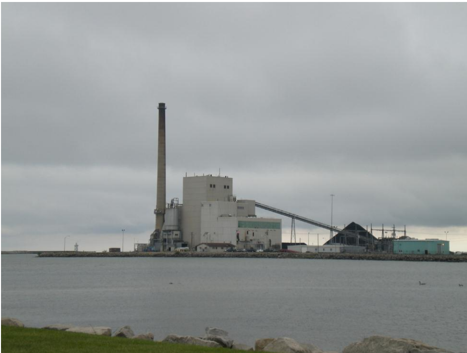
Figure 3.3: DTE's Harbor Beach Generating Station
