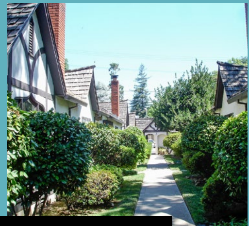
Examples of the Bungalow Court building type.
