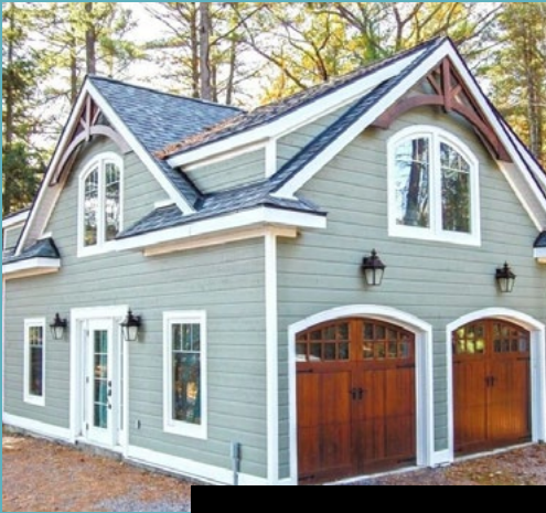
Examples of the Carriage House building type.
