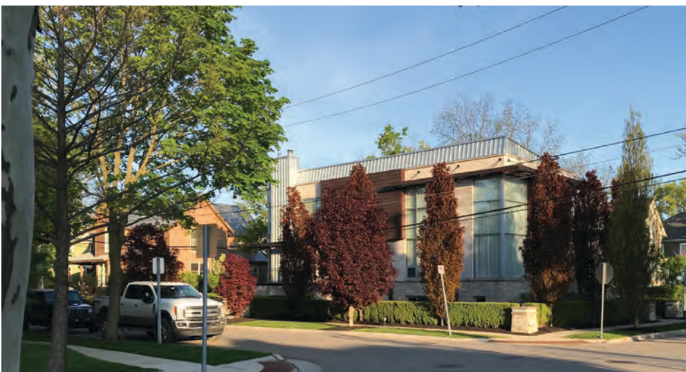
Figure 43. High quality contemporary infill, in scale with neighborhood fabric.
