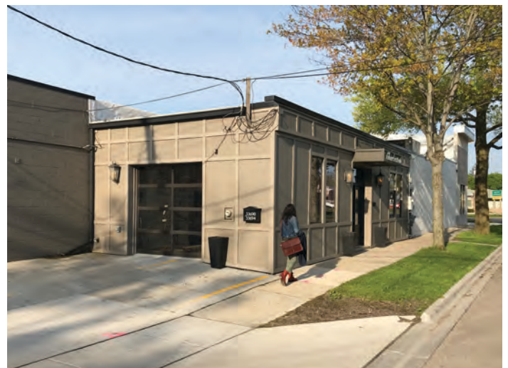
Figure 54. Building with potential for sleeve activation.
